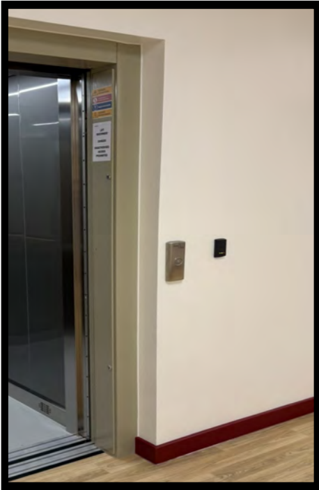
Optional lift control interface to enable restricted use of landing control panel by authorised persons *
