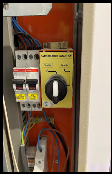
Optional card/fob isolation switch to enable unrestricted use of the lift
