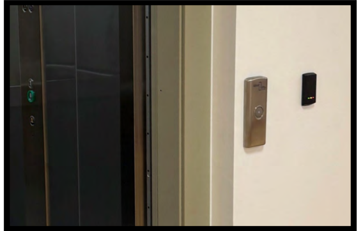
Optional lift control interface to enable restricted use of landing control panel by authorised persons *
